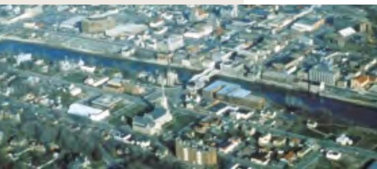
Encroachment of the floodplain
